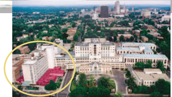
The new home of the Comprehensive Women's Health Center at Saint Francis is conveniently located at the former site of the Hospital's Emergency Department.
